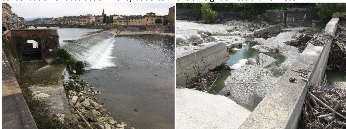
Left: consolidation weir (Arno river, Italy). Right: retention check dam (Marecchia river, Italy). Pictures: S. Bizzi (left), B. Belletti (right)
