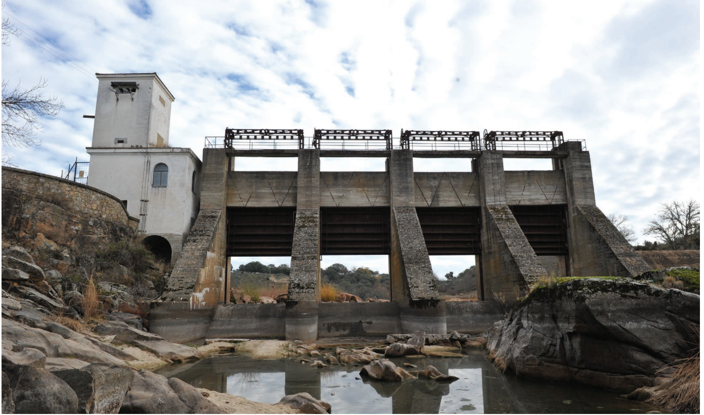
The Yecla de Yeltes Dam in Spain is being demolished in the largest project of its kind ever in Europe.
