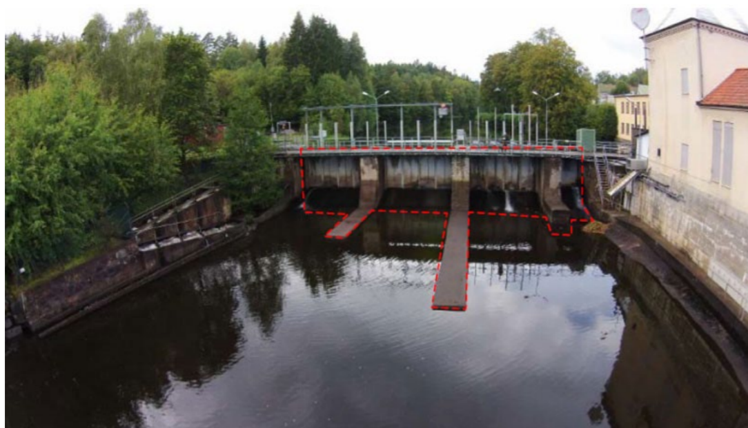
The Marieberg Hydropower dam, dotted line shows which parts will be removed.
