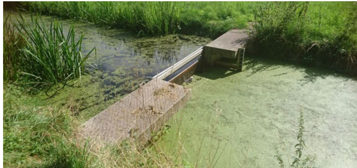
Small weir in the Netherlands
