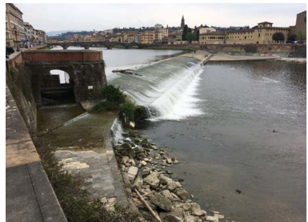
Consolidation weir (Arno river, Italy). S. Bizzi (2017)
