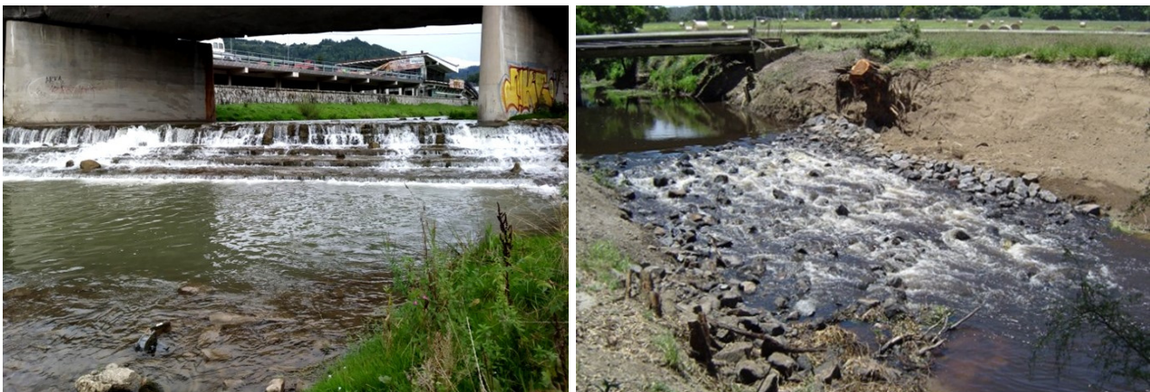
Figure 7. Examples of a ramp under bridge (left) and mitigating solution (right) (photos: Z. Kaczowski, SSIFI; AMBER).
