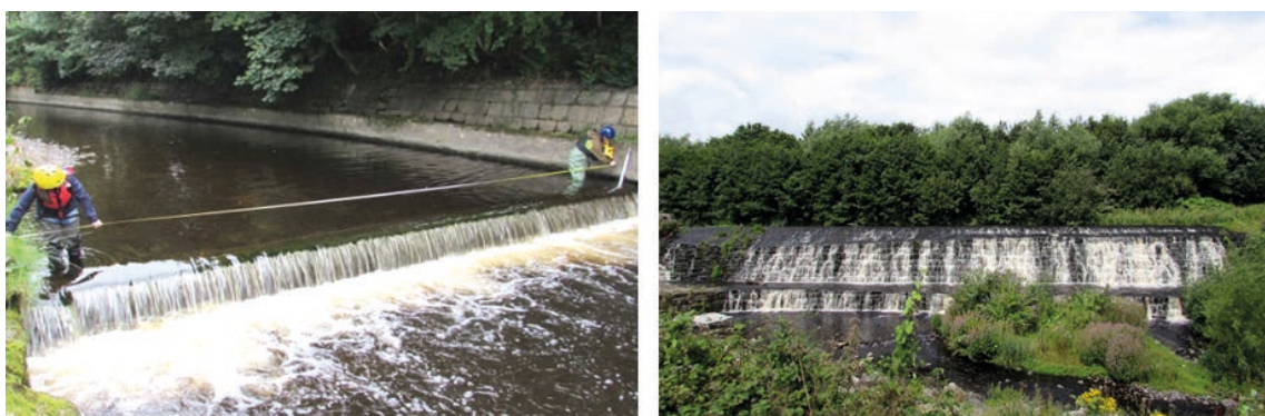
Figure 3. Examples of overflowing weirs (photos: I.Wagner, ERCE; K. Suska, SSIFI, Poland).
