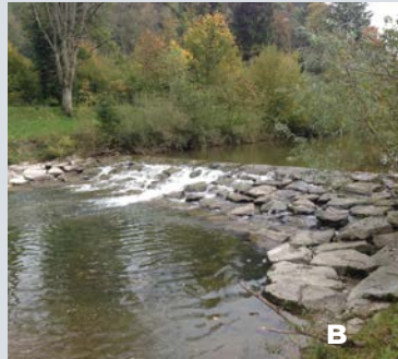
A) Bed sill (Marecchia river, Italy). B. Belletti (2017) B) Rock ramp (Switzerland). R. Bösiger (2018)
