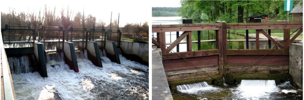
Figure 4. Examples of sluice gates (photos: Z. Kaczkowski (ERCE; Polish Waters Warsaw)).
