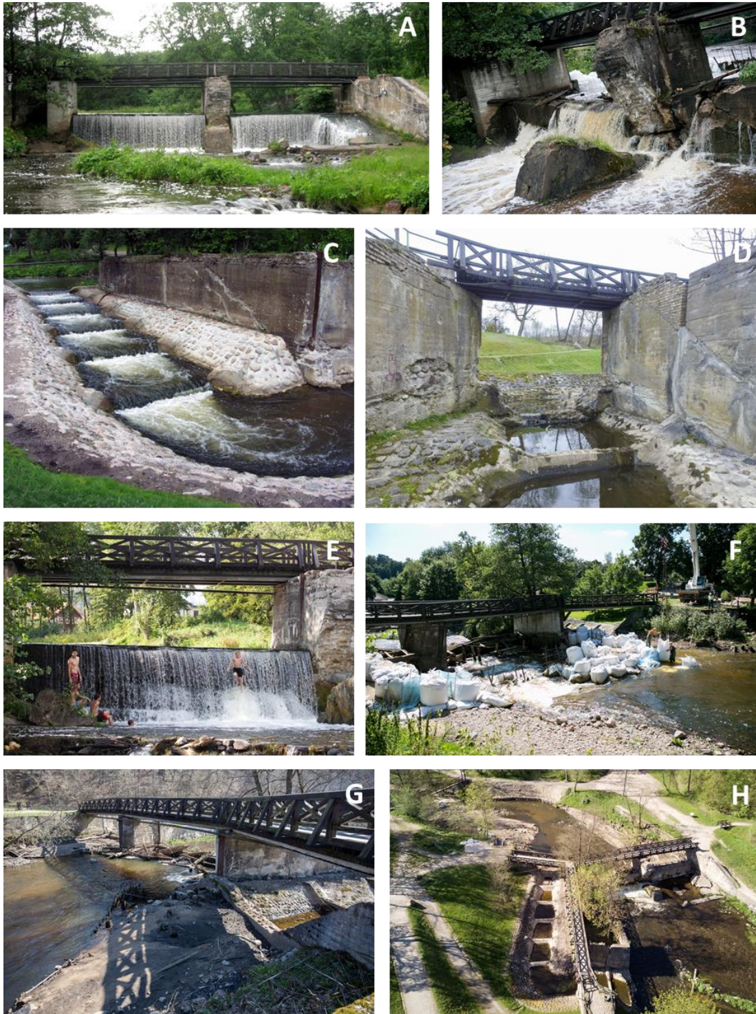
Figure 8. Belmontas dam before (A) and after (B) the collapse; the fish ladder before (C) and after (D) the collapse; the “waterfalls”, known to attract tourists, before (E) and after (F) the collapse. View from upstream (G) and aerial view (H) of the dam after collapse.
